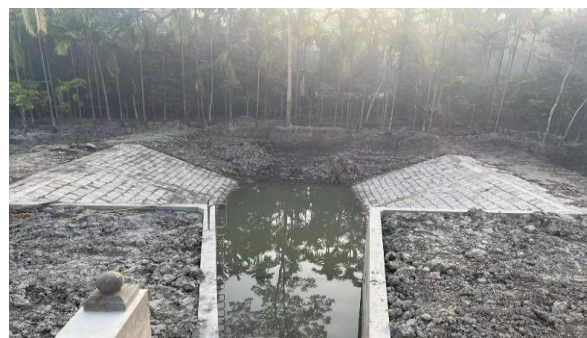
Figure 3-27: Sluic Inlet-Outlet Placing cc block for FS-14 in Polder-39/2C
