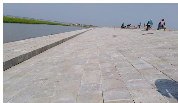
Figure 3-10: Completed Slope Protection Works in Polder-32
